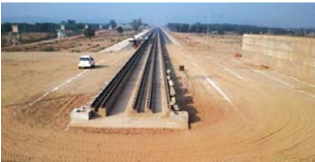
Side View of the Augmented RTRS Facility
